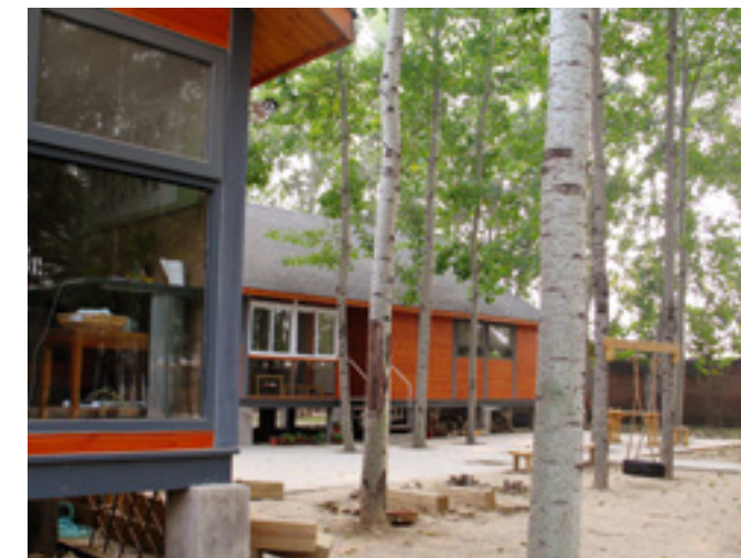
School building at Zhong Guan Cun Waldorf School
